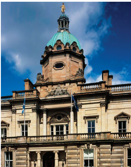
Bank of Scotland Head Office
